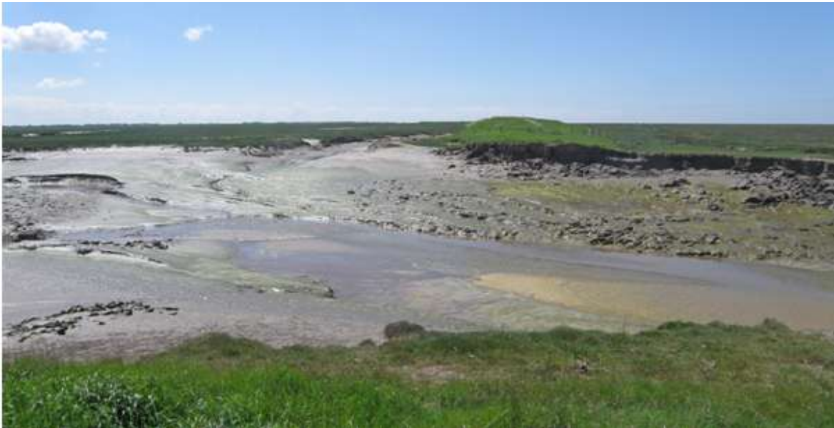
Figure 2. Breach at Hesketh Outmarsh, one of the main areas within the site that is likely to form sustainable inter-tidal sandy and muddy habitats
