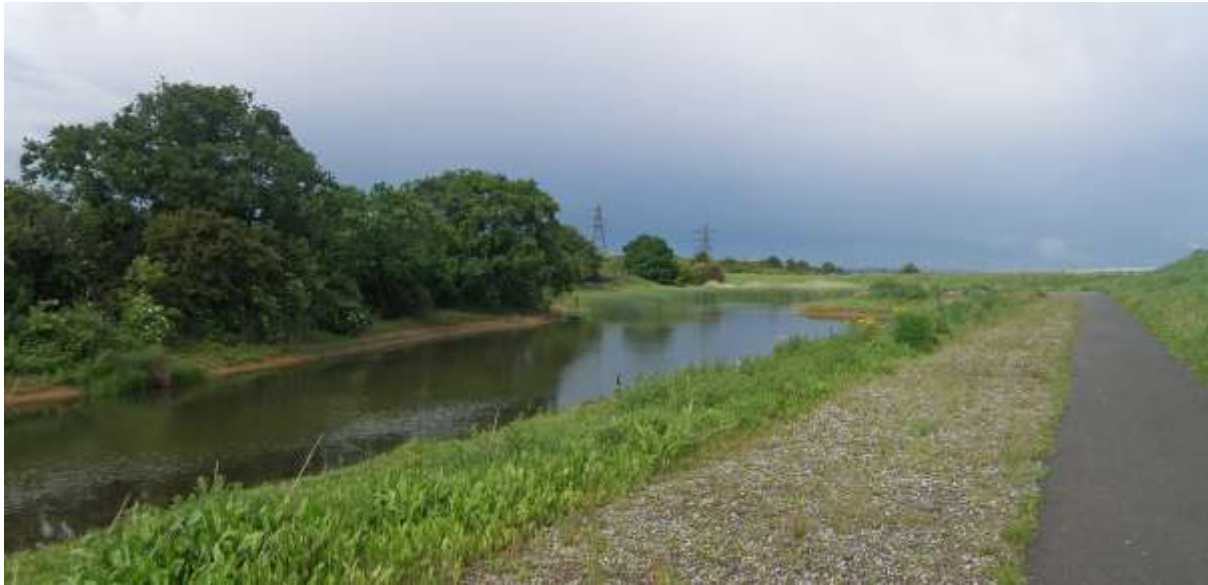
Figure 6. Borrow-dyke and disabled access surface at Stanford Wharf (Mucking) (Site A): an example of good design practice that makes use of an engineering feature to provide wildlife, landscape and public access benefits.
