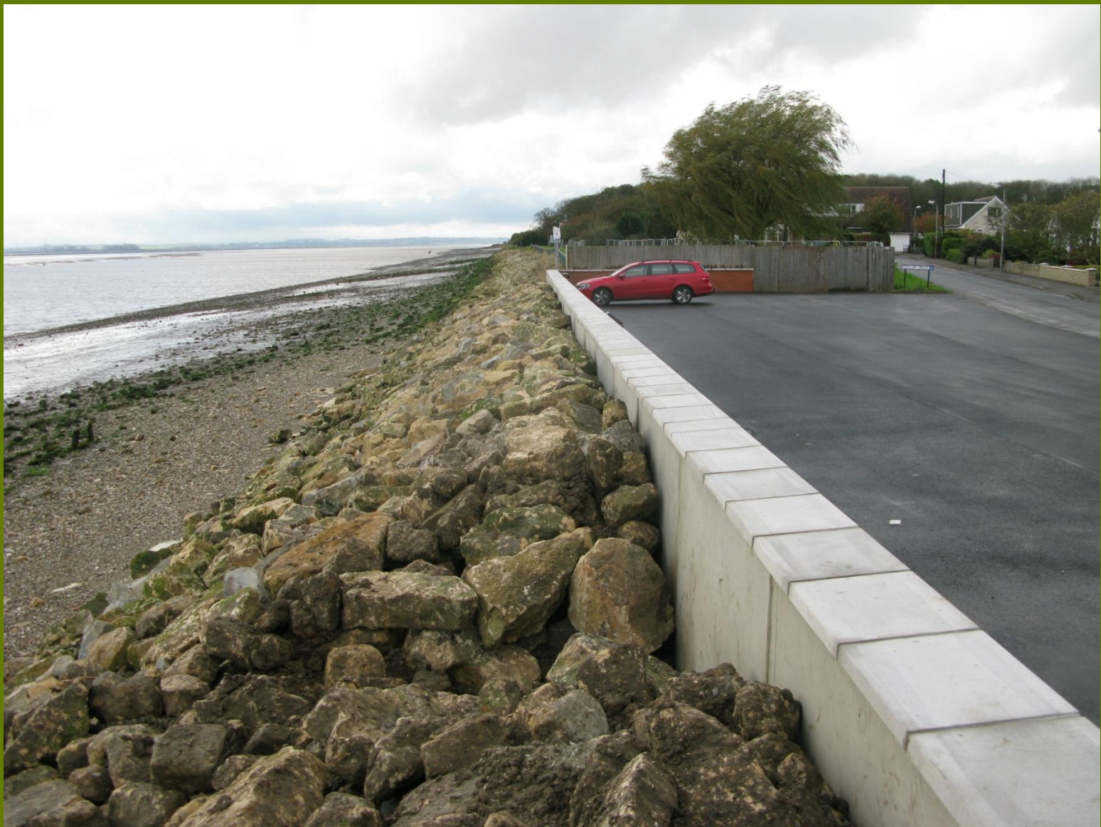
North Ferriby showing works completed to date. Further work now underway.
