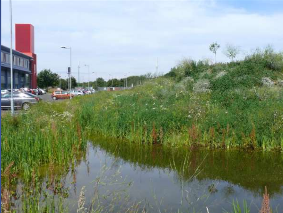
Hull KR Stadium SuDS – July 2014
