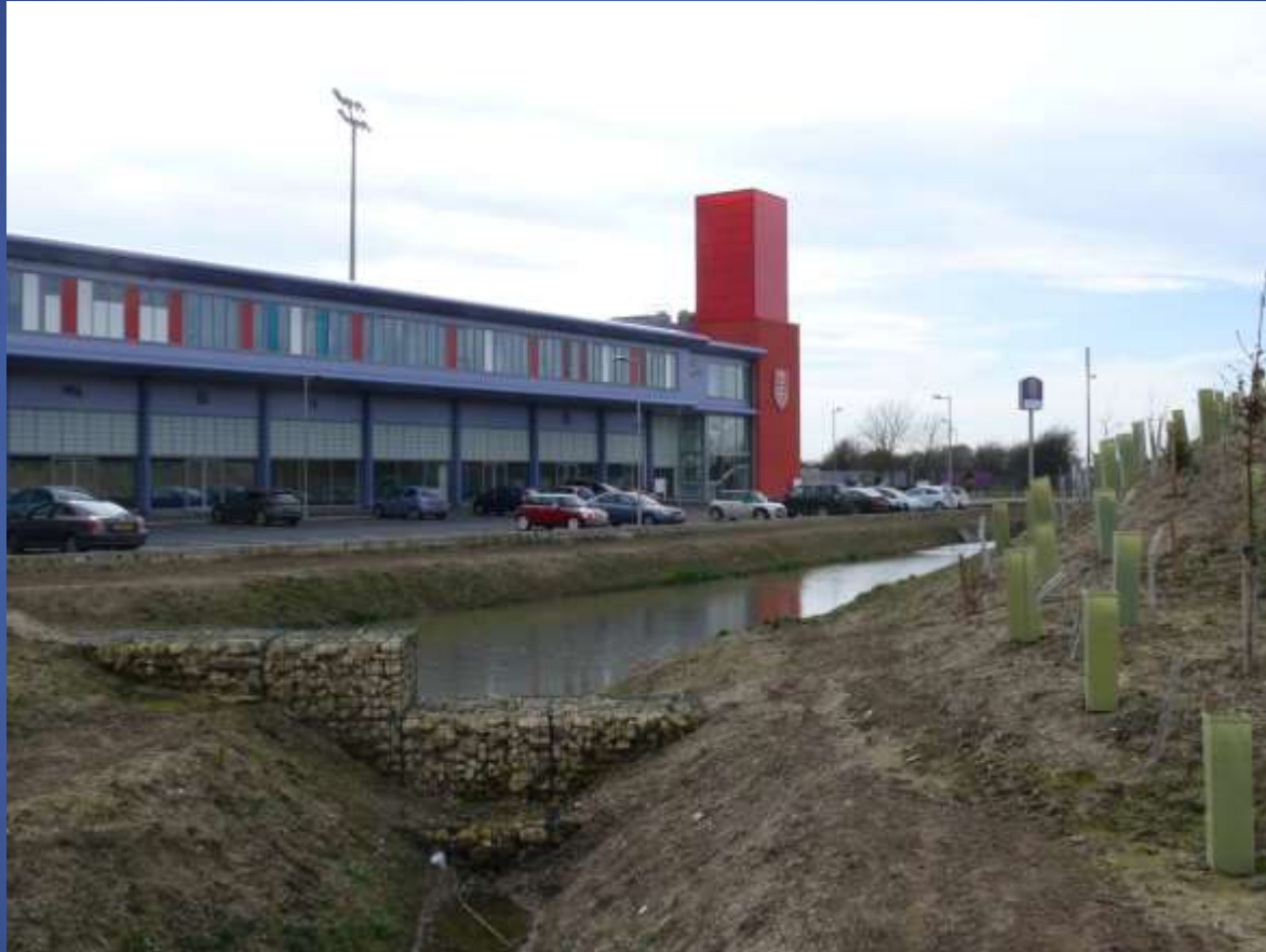
Hull KR Stadium SuDS – March 2014
