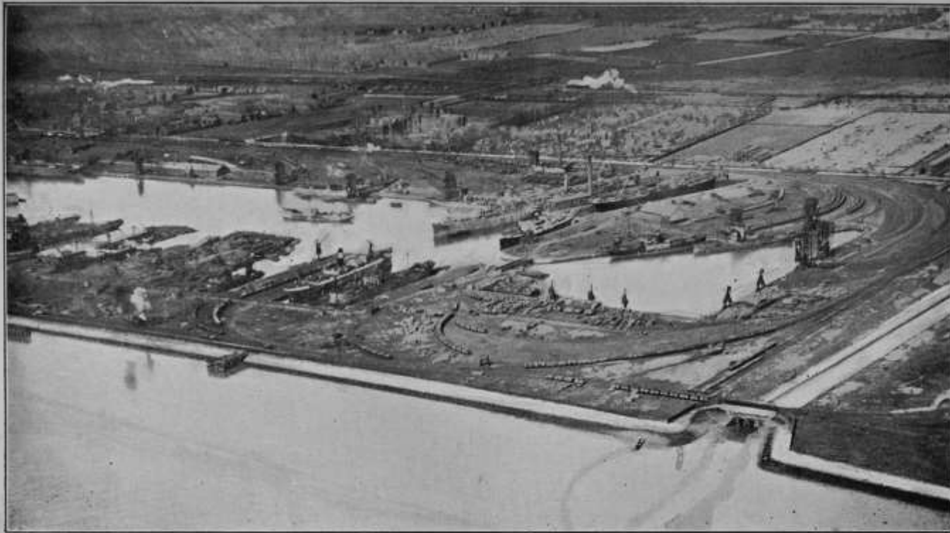
THE ALEXANDRA DOCK, HULL.
