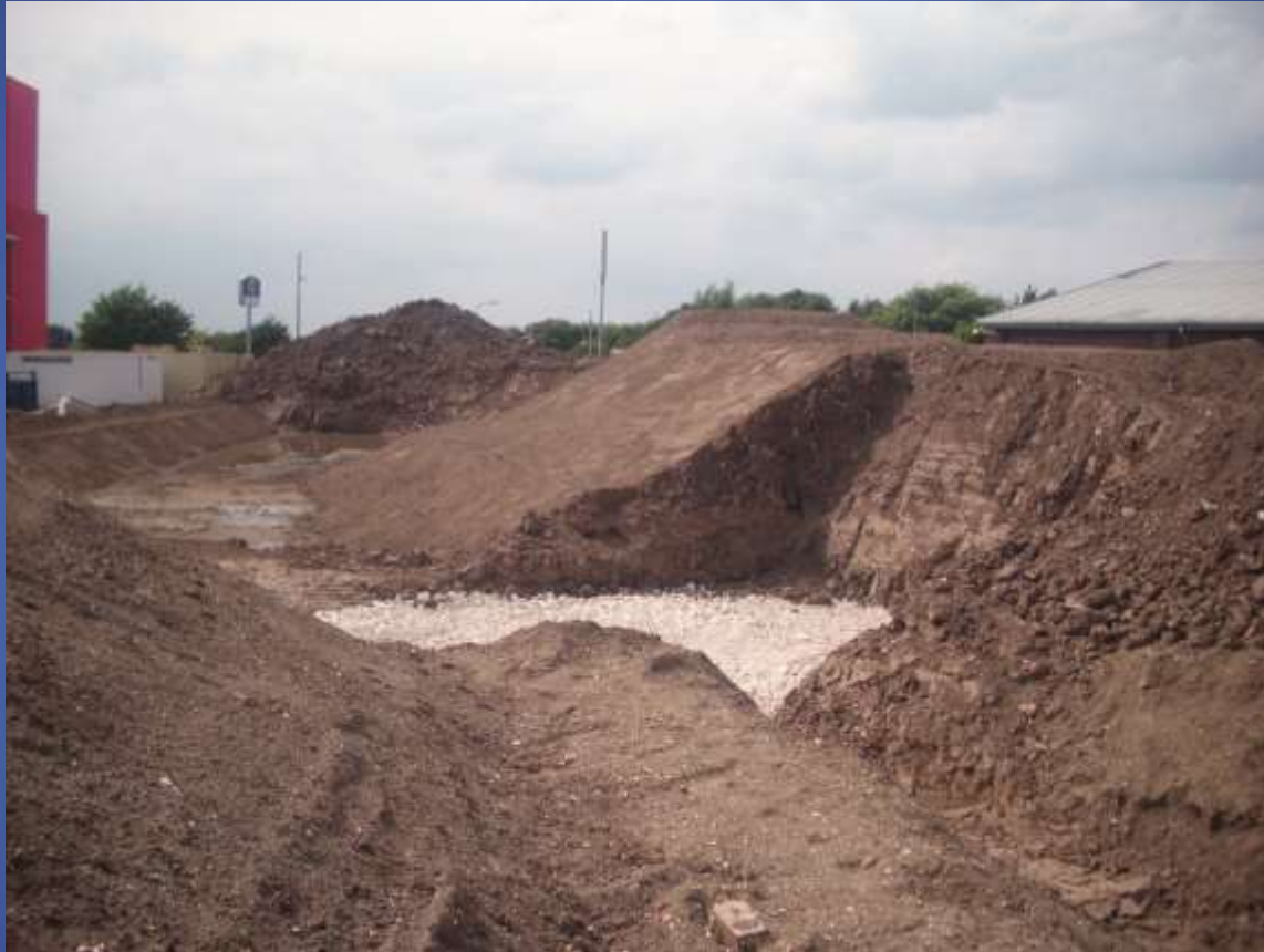
Hull KR Stadium SuDS – August 2013
