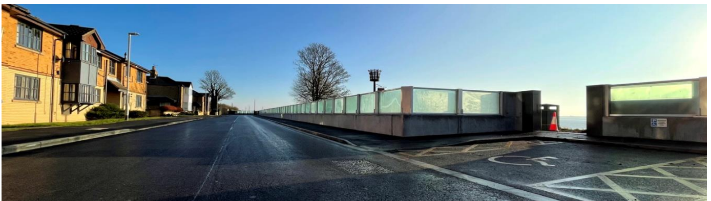
Fleet Drain Sluice; A63 Barrier; Cliff Road Defences
