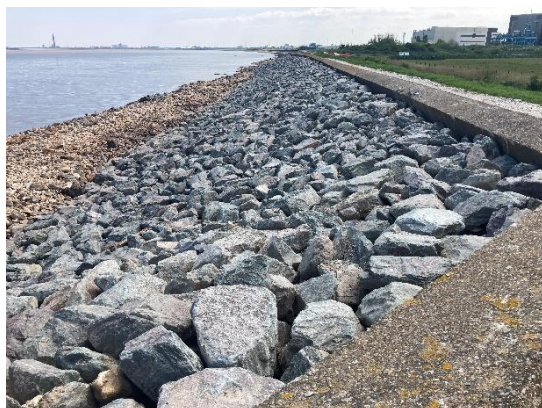
New rock armour installation
