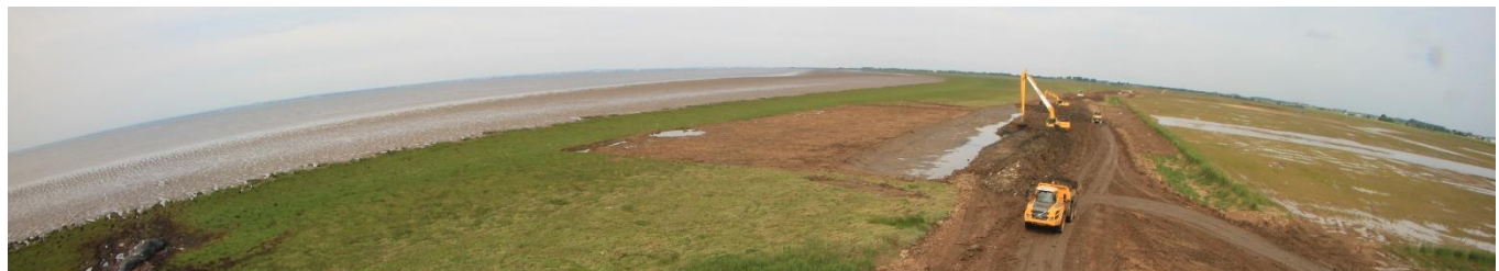
On going breach work
