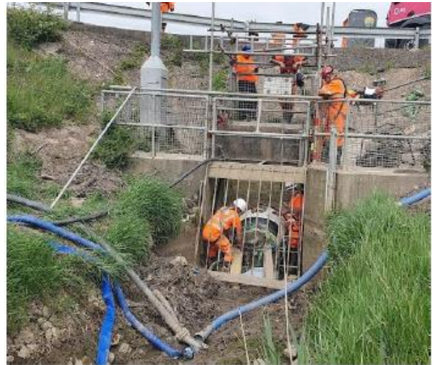
Slip liner installed through outfall
