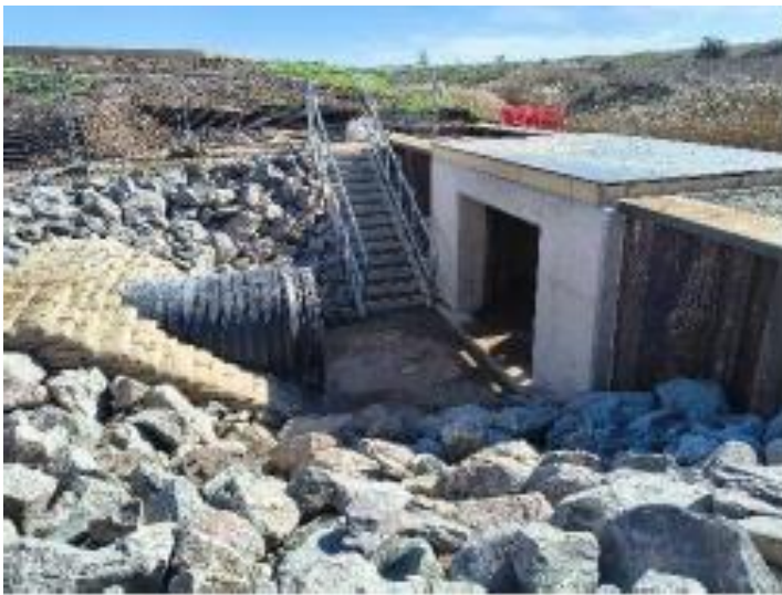
New overflow structure
