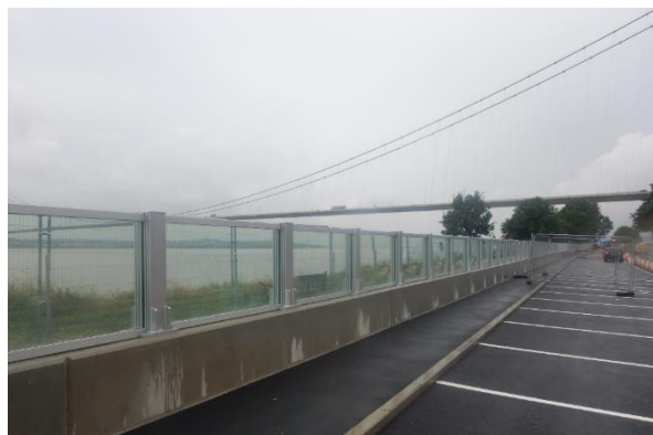
Stage 3 Wall progress showing installed glass panels
