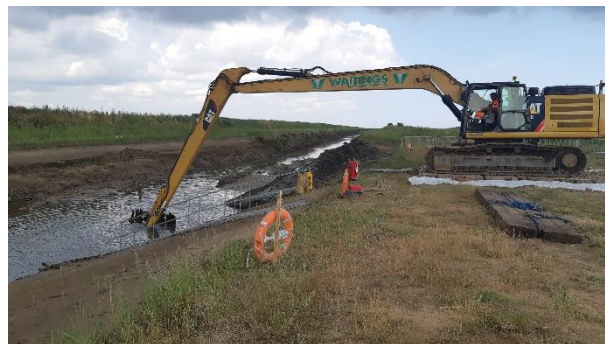
Piles being removed
