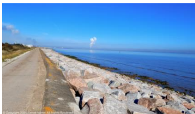
Granite rock armour to 3km of the coastal flood defence
