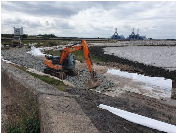
Oldfleet Drain access track construction
