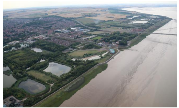
View of Barton-upon-Humber estuary frontage looking west
