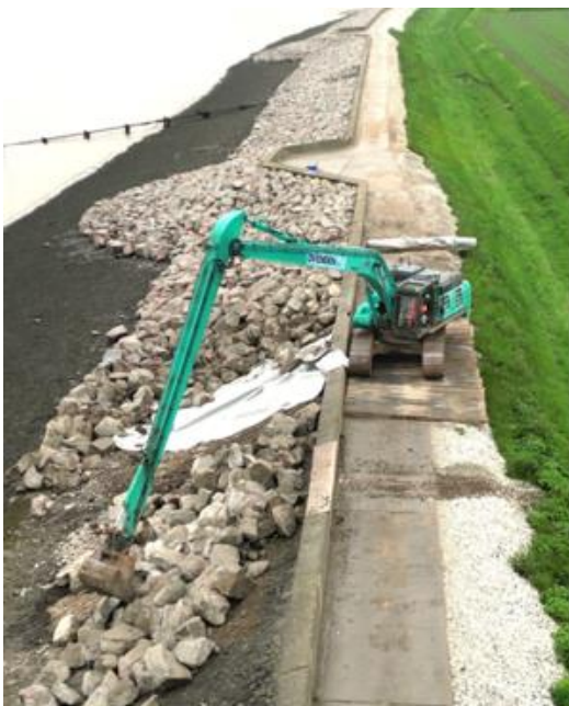
Section 1 rock armour installation
