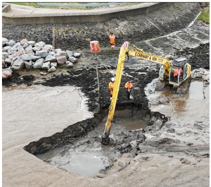
Oldfleet Drain desilting
